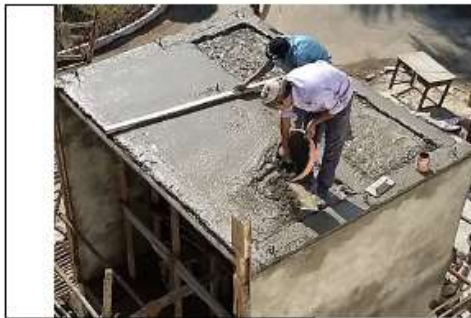
Fig. 3 Spraying and pouring of concrete over the EPS core skeleton and finished building model
