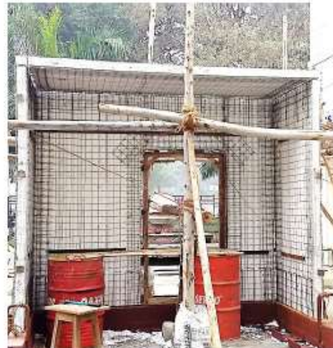
Fig. 2 Building skeleton made of factory made EPS core panels
