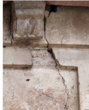
CRACKING ■ ■ ■ Formation of fissures in the structure. Caused by- Structural inheritance
