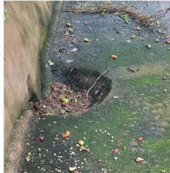
MOSS GROWTH ■ Green fuzzy stuff that appears on the roofs and buttresses. Caused by- Stagnant water and moisture.
