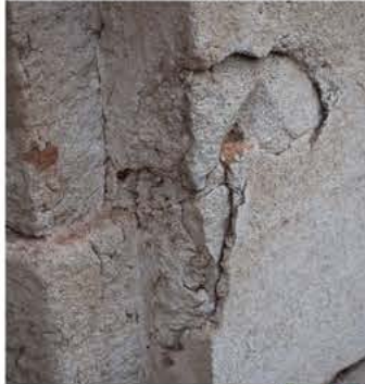
PEELING OF STONE ■ ■ ■ The surface of the stone flake or peel away. Caused by- Weathering or improper application of mortar.
