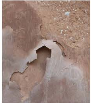
BLISTERING OF SAND- STONE ■ Swelling and rupturing of wall skin. Caused by- De-icing salts and ground moisture.
