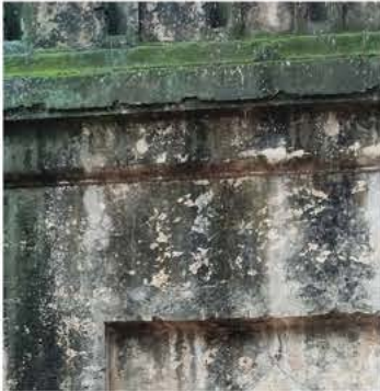
MOSS ON PARAPET ■ ■ A green plant that is visible on the buttresses and parapets. Caused by- Absorption of rain and water.
