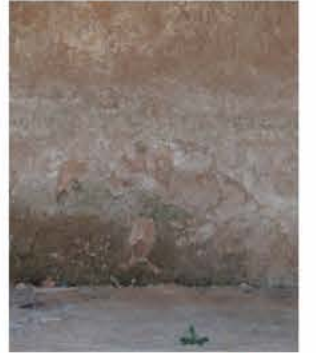
EFFLORESCENCE ■ A whitish haze is visible on the walls. Caused by- Entry of water into the structure.
