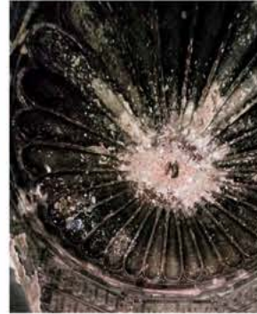
DEGRADING OF STONE CEILING ■ The ceiling of the tomb has darkened. Caused by- Contact with air and moisture over the years.
