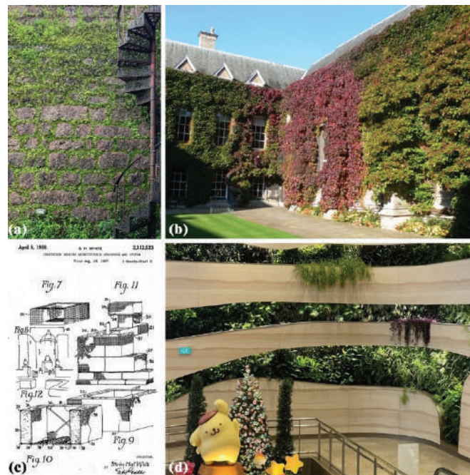
Fig.1. Historical progression of vertical greenery systems. (a) Spontaneous growth of mosses and lichens on masonry walls at Reis Magos Fort, Goa, India (Image: Author); (b) Ivy covering the Front Quad of Lincoln College, Oxford, where climbing plants have been recorded since the 1860s (Image credit: Rémi Mathis, Wikimedia Commons, licensed under CC BY-SA 3.0); (c) Stanley Hart White's 1938 "botanical bricks" patent drawings (US Patent No. 2,113,523, public domain); (d) Living walls designed by Patrick Blanc inside the Changi International Airport, Singapore (Image: Author).
