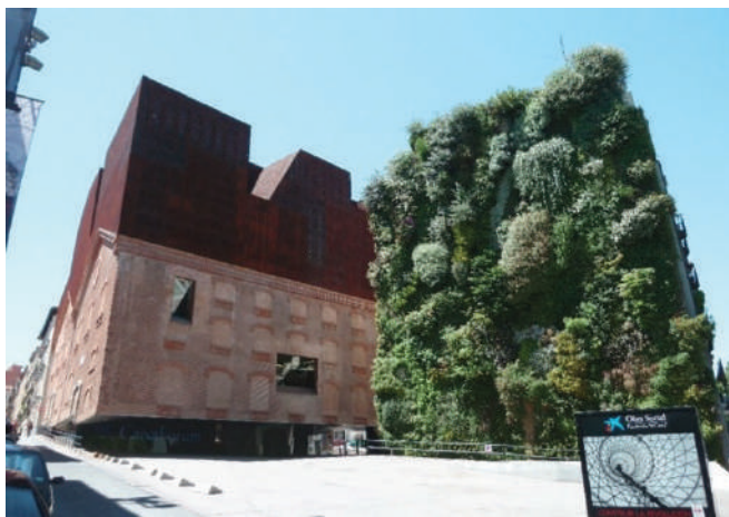
Fig.5. CaixaForum Madrid. Continuous hydroponic living wall applied as an urban vertical greenery system adjacent to a cultural building. Image credits: Wikimedia Commons, licensed under Creative Commons (CC BY-SA).
