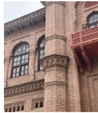
Fig. 4. Use of exposed brickwork and sandstone in façade Source: Authors
